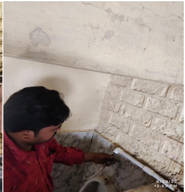
Toilet minor repair Works
